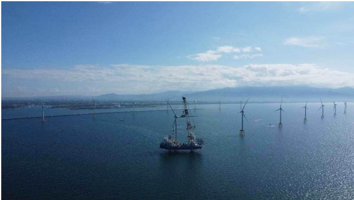
Last turbine installation
